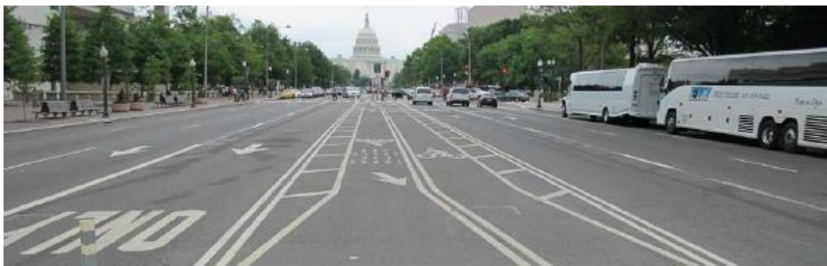
**Figure 18. Median buffered bike lanes, Washington, D.C.**
