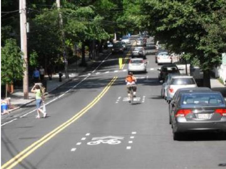
**Figure 63. Sharrows with dotted lines as evaluated in Brookline, Massachusetts.**
